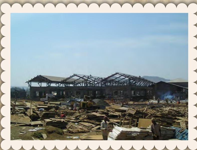
May 6th, 2006, the workshop, which is sitting upon red volcanic basalt rocks featured three bays and a factory-like roof, ensuring ventilation for student work. Its uniquely designed roof, requiring extra budget and 20 MT of structural steel, now supports solar panels, promoting green energy.
